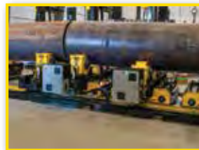
Sections brought together using powered track drive
