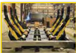
Hydraulic alignment jacking system to align and pull vessel sections together
